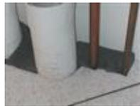
to make any size or shape needed. PolarDAM Air Dam Foam sheets are 24" x 24" and 2 inches tall and each box has six sheets, or 24 square feet of foam. Simply cut off the size you need and stuff into the floor opening. Works great to fill miscellaneous gaps in racks, too!
